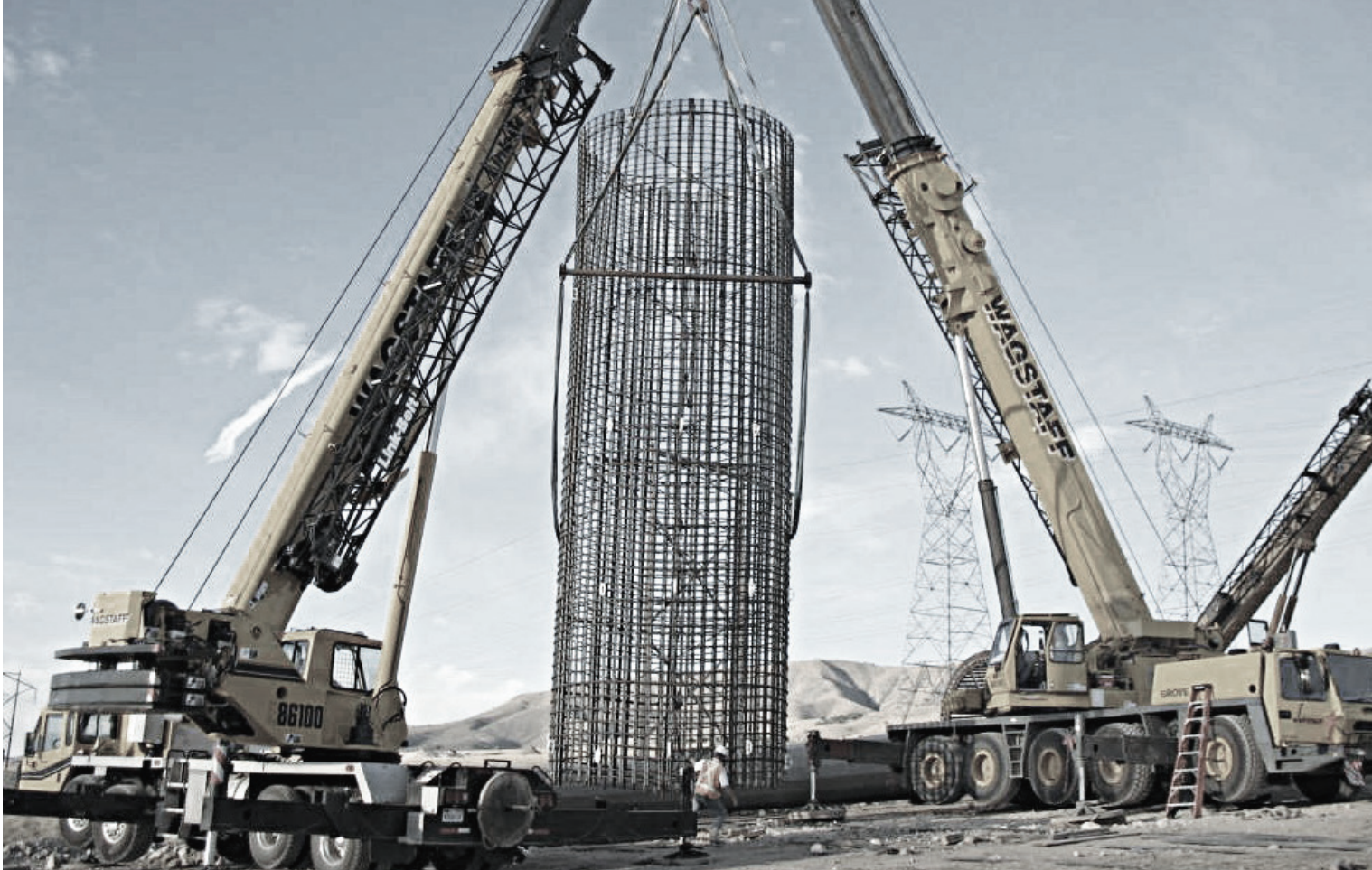
ShaftSpacers attached along large-diameter reinforcing cage
