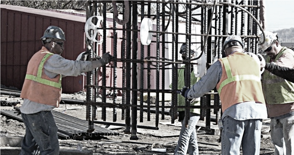
Guiding rebar cage into drilled shaft with ShaftSpacers attached
