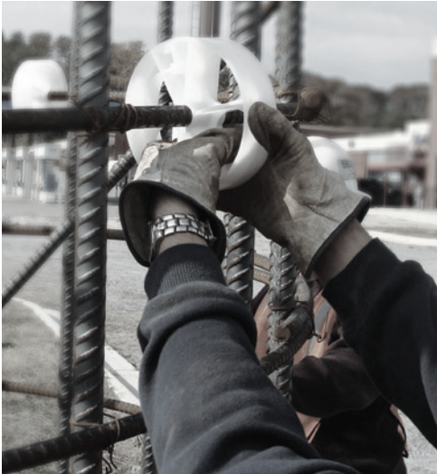
Installation of ShaftSpacer
